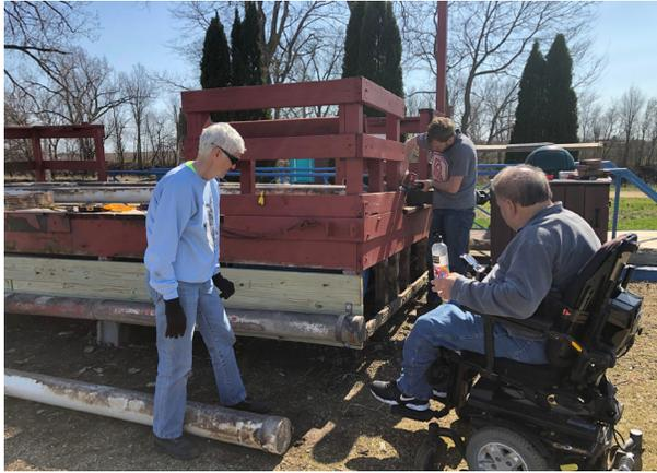
After about eight years of use, the floating dock at McConnell needed repair. The boards at the lower structure, on four sides, were recently replaced. Lee Butler stands next to floatation added to the Wes Block floating dock.
